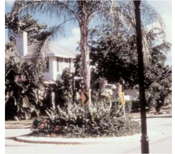
Traffic calming devices, like this traffic circle, slow down traffic and are aesthetically pleasing.
