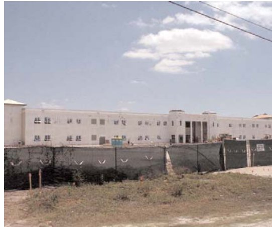
Tradewinds Middle School (Under Construction)
