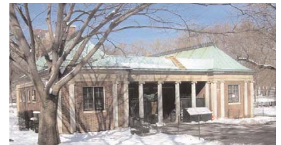
Park Pavilion in Central Park: Built in the great tradition of beautiful park structures
