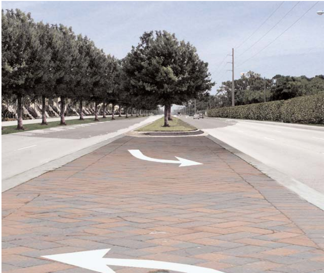
The final buildout of Military Trail includes a new brick paved turn lane, hedges hiding the Atlantis Wall, new street streets, and beautiful townhouses on the western side of the road.
