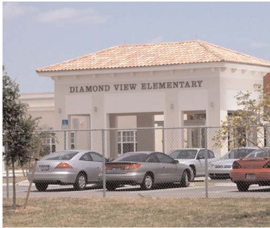
Diamond View Elementary School
