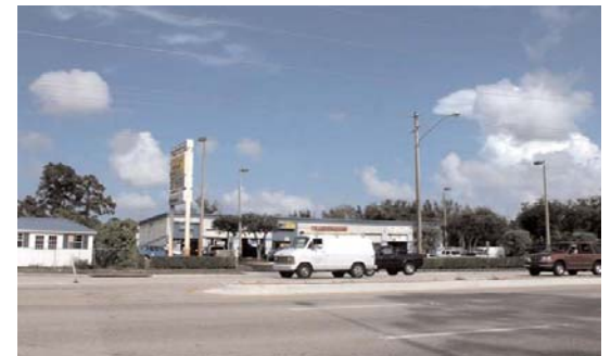
Existing commercial buildings on Military Trail
