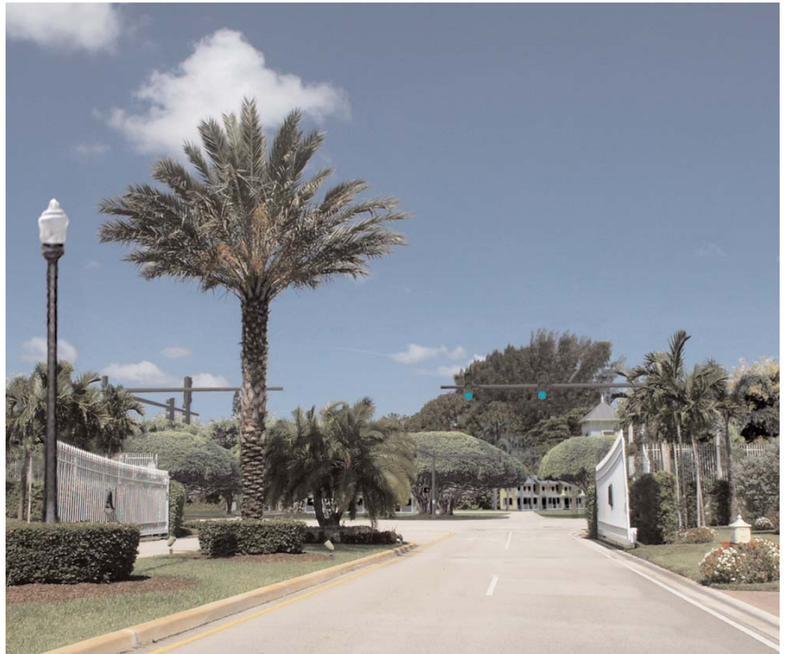
Final buildout: The new traffic signal will make left turns from Atlantis safer, provide for a future four-way intersection, and will also calm traffic on Military Trail.
